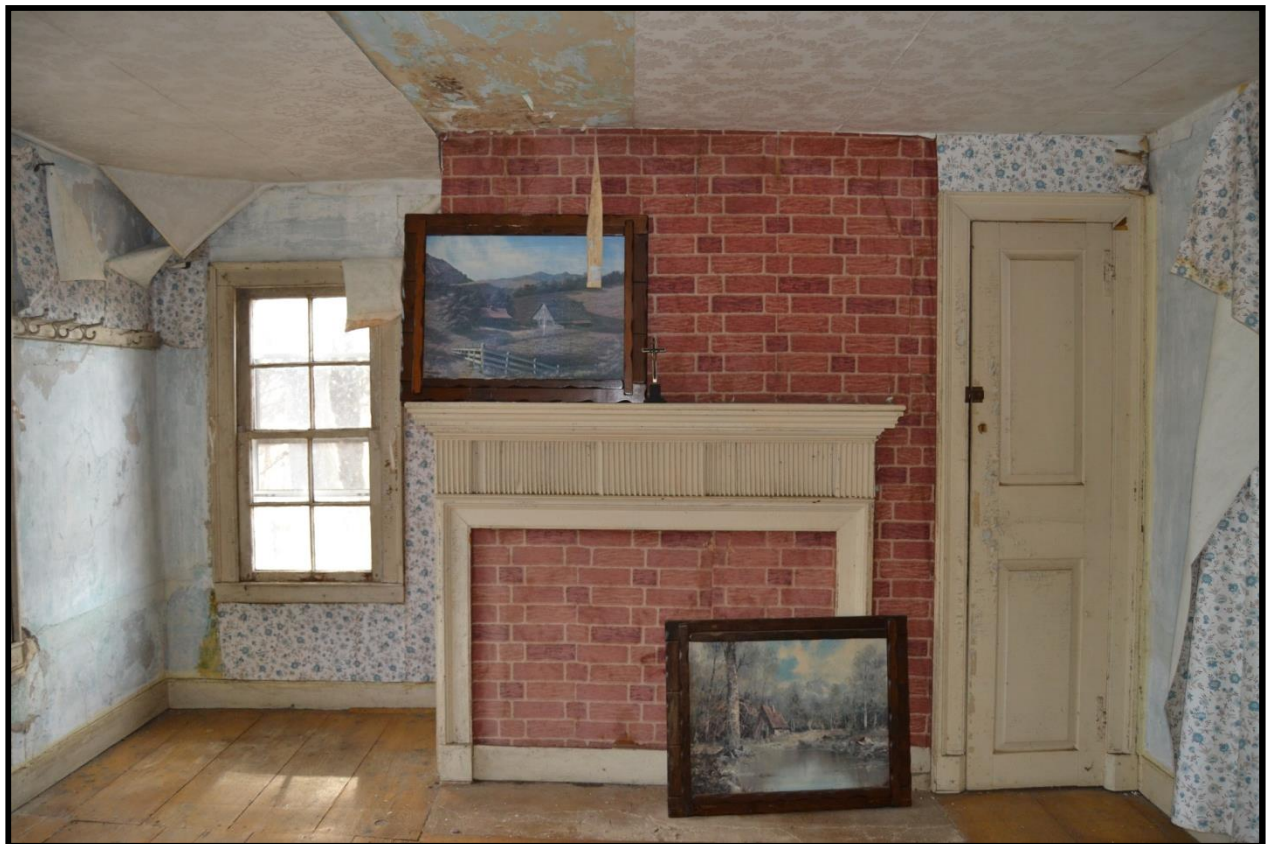
Figure 8: The Federal style mantel of the 1798 Mount Lubentia in Prince George's County, Maryland (HABS MD,17-LARG) is a more elaborate version of the reeded and paneled mantel constructed by Obadiah Buckelew, below.
