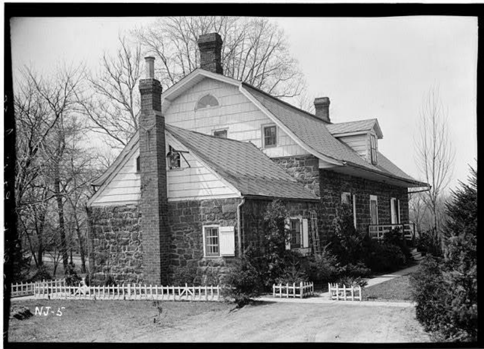
Figure 5: The smaller wing of the Zabriskie-Christie House in Dumont, Bergen County was the original house, likely built in the mid-18 th century. Aside from the different building materials, it is similar to the house the Buckelews built with its 1 ½ height, steep roof with minimal eave and asymmetrical fenestration. HABS NJ,2-DUMO
