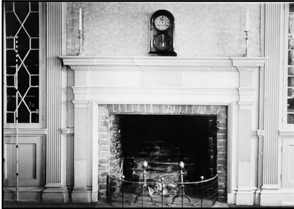
Figure 8: The Federal style mantel of the 1798 Mount Lubentia in Prince George's County, Maryland (HABS MD,17-LARG) is a more elaborate version of the reeded and paneled mantel constructed by Obadiah Buckelew, below.
